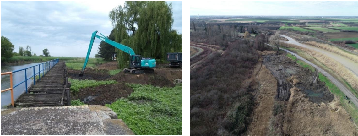
Figure 5-2. Sediment dredging and aerial view of disposal site (2017)
