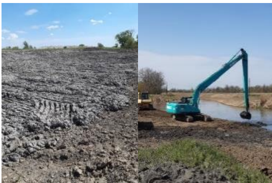
Figure 5-4. Dredging and deposition of sediments at Landfill 2
