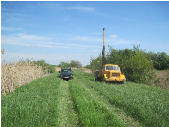
Figure 5-3. Construction of piezometers for groundwater monitoring (2017)
